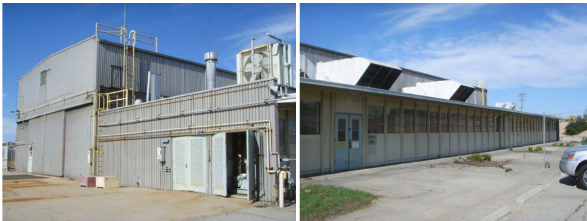
(southeast end of building; view from south corner)
